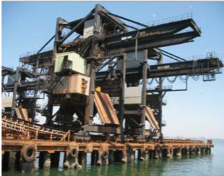
Figure 32. Tyres abutting jetty when filled with rain water can be extremely dangerous in providing the first foothold to any mosquito arriving with a ship © Ashwani Kumar
